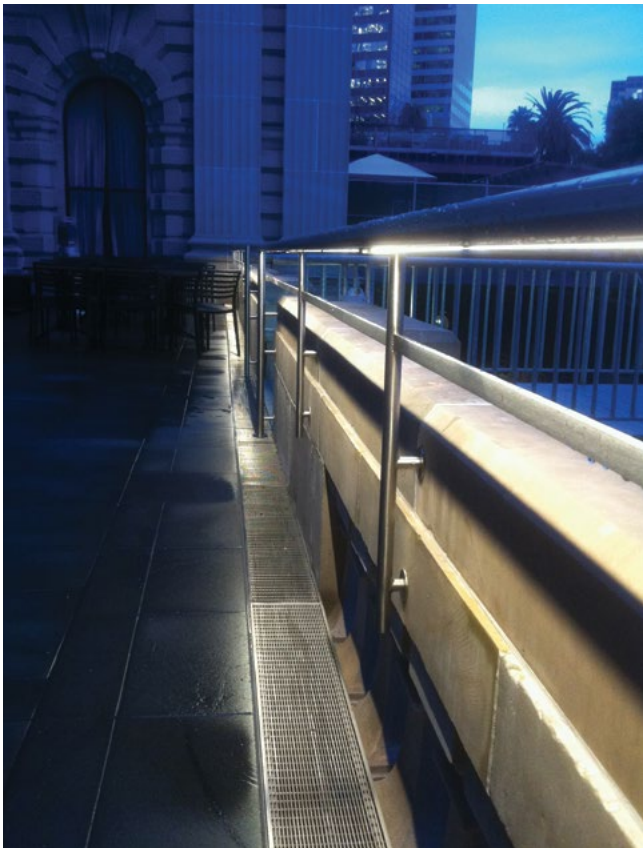
The illuminated new handrail highlights the stone balustrade whilst providing after hours lighting across the terrace
