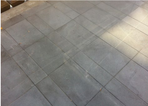
A section of bluestone paving on the east terrace, almost complete
