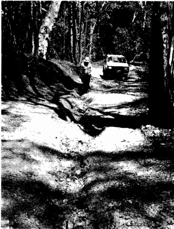
(Left) A deeply guttered and washed out track in the Alexandra region.
