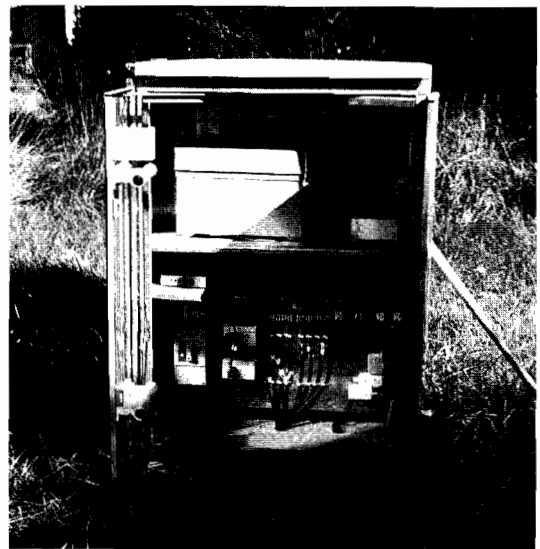
A STEP permanent traffic recording station. The hourly volumes of cars, trucks, and semitrailers are recorded for transmission to head office over the telephone system. About $130,000 a year is saved with this system.
