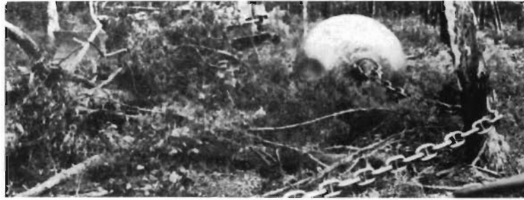
Clearing operations at Heytesbury.
