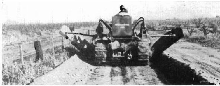
Constructing deliver channels on irrigation project.
