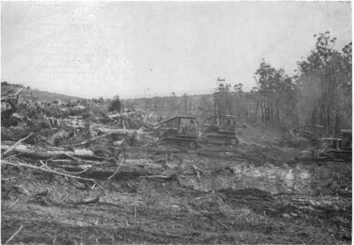
Windrowing operations on the Heytesbury Project.
