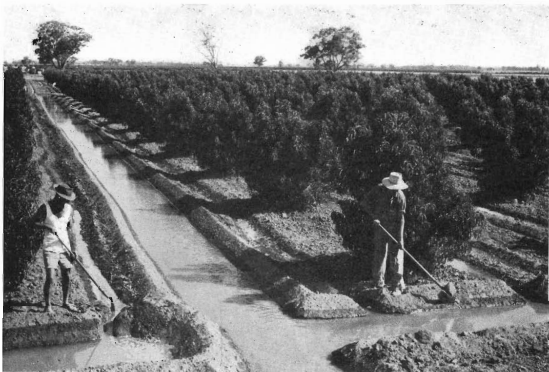
Irrigating an Orchard Holding at East Goulburn.
