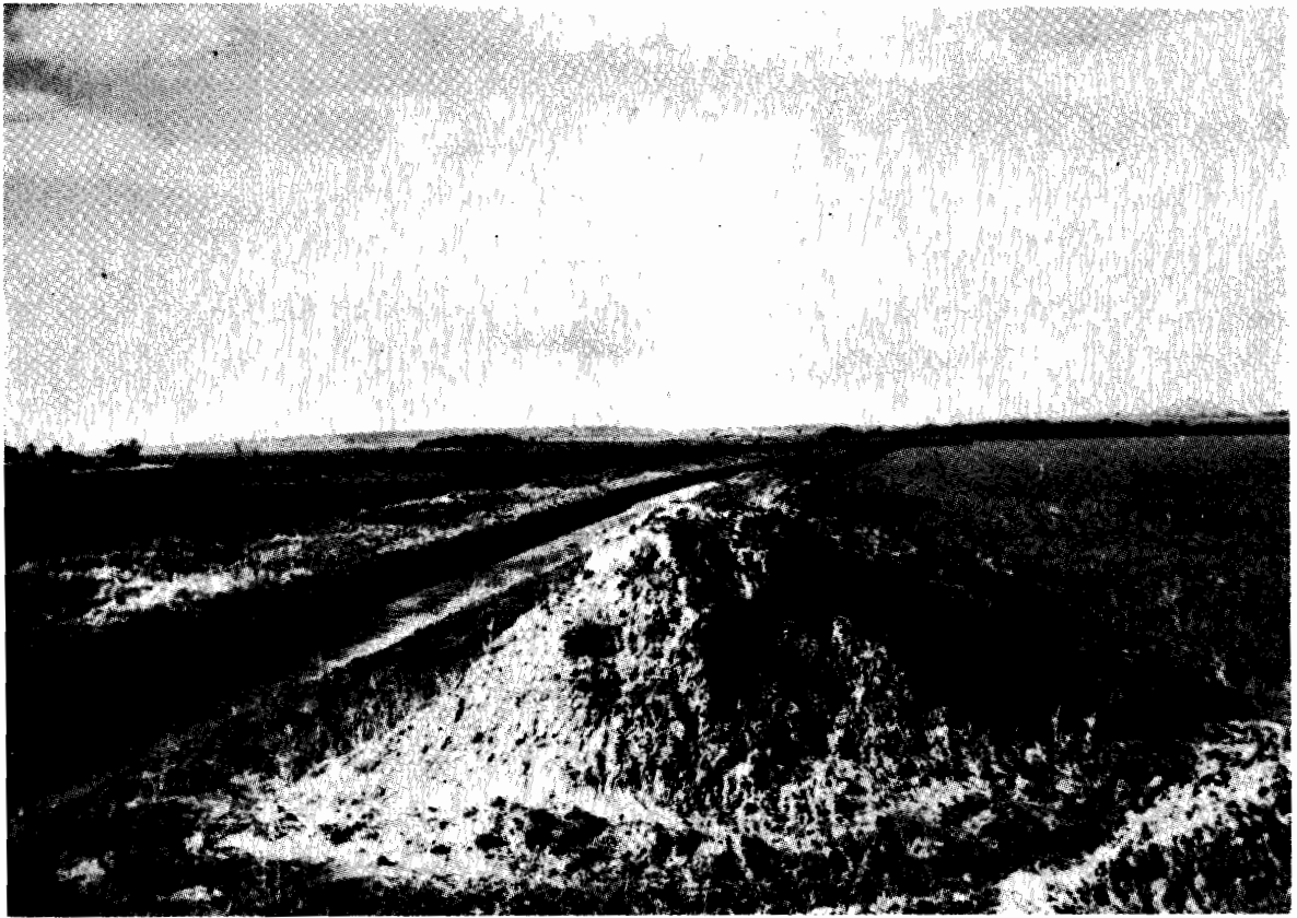
Portion of the drainage works carried out on the Swamp Area at the Yanakie Project.
