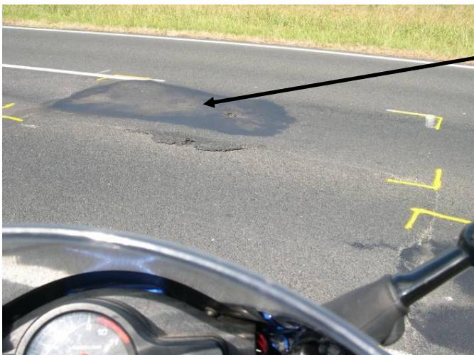
About an 80mm difference in the road surface. This can cause a motorcycle to be moved off line or cause problems when braking.
