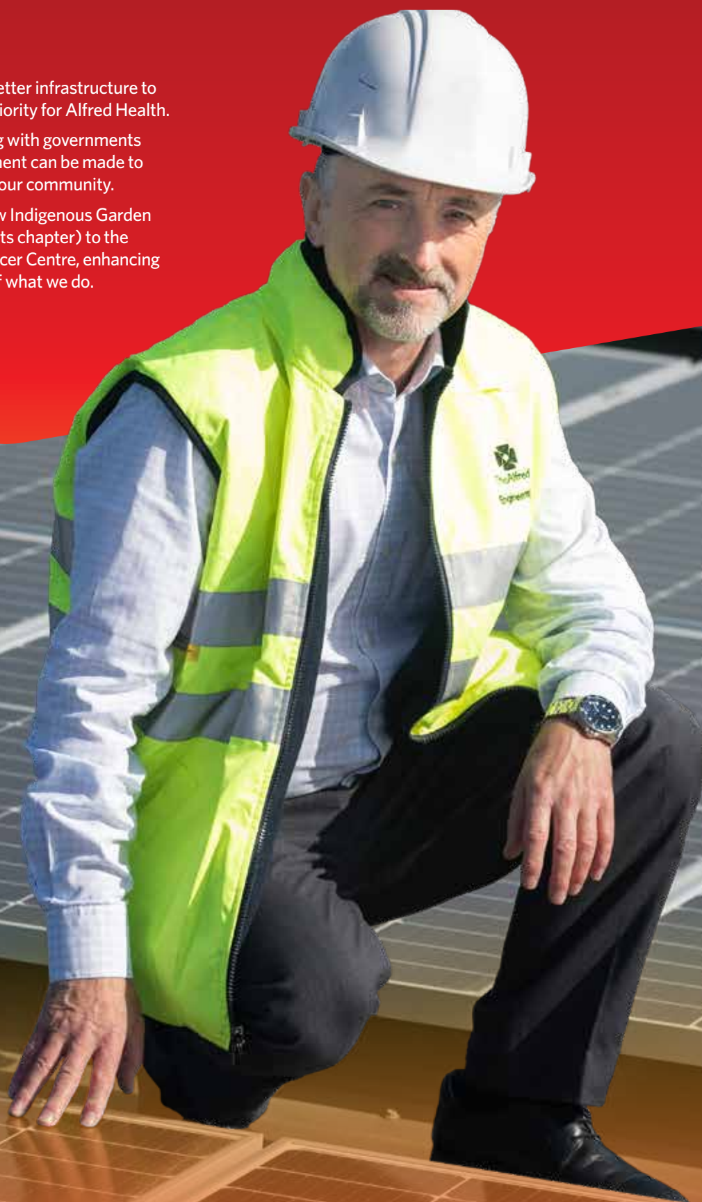
Deputy Director of Engineering & Facilities Caulfield, Sandringham and community sites Jim Hamilton with the new solar panels at Caulfield hospital.
