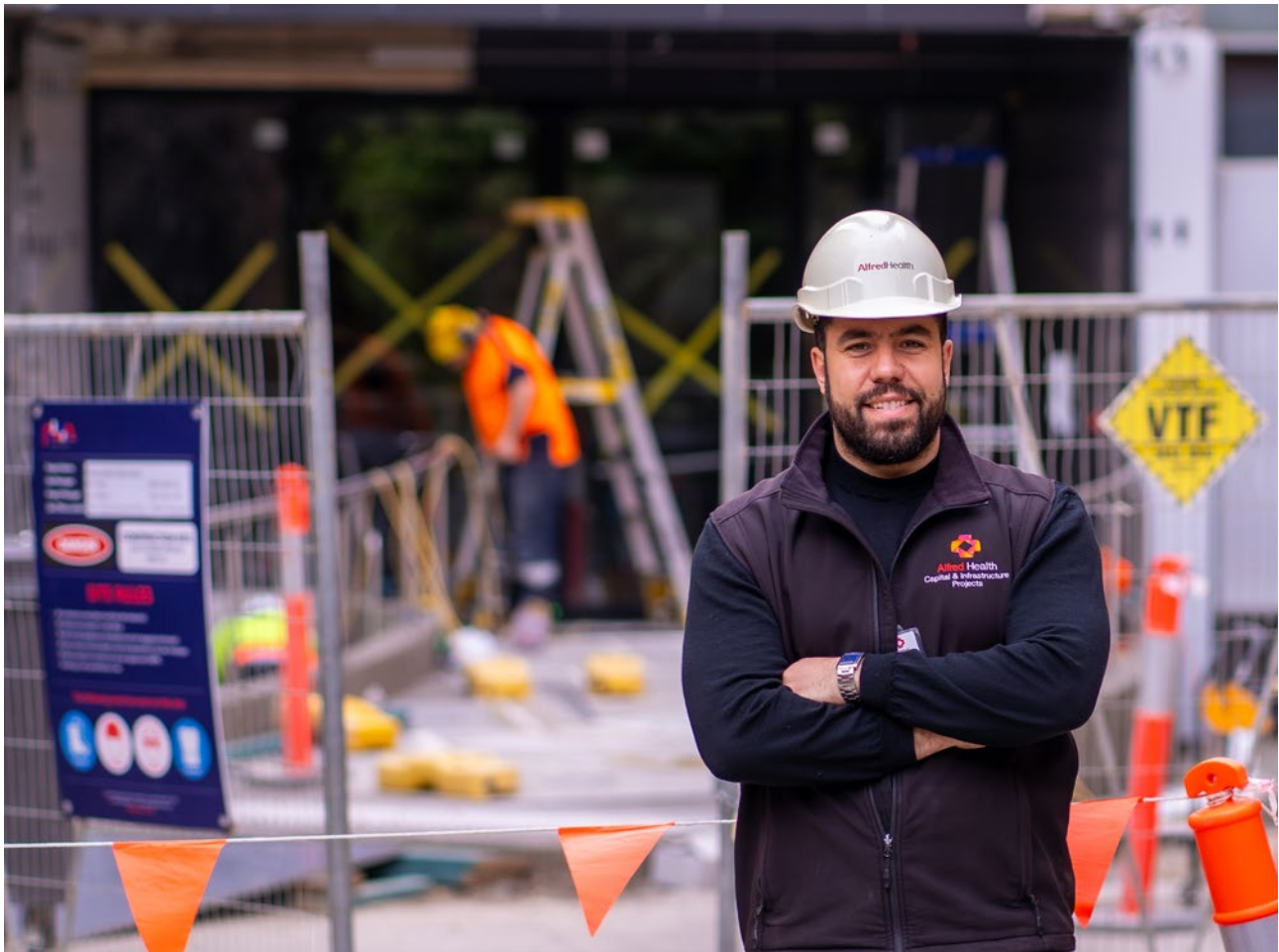
Fresh look: Capital and Infrastructure Project Manager, Steve Skapetis, is leading the team working on The Alfred's new Retail Precinct.
