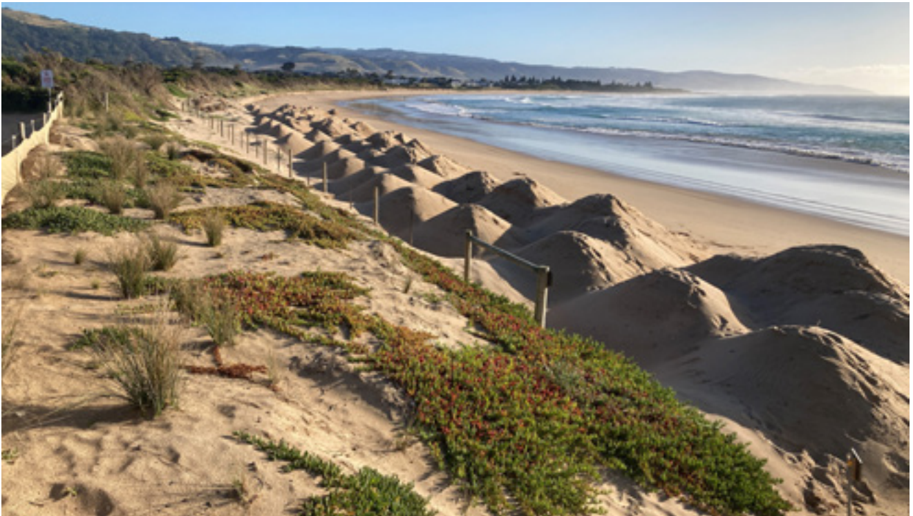
Beach nourishment works at Mounts Bay facing Point Bunbury.
