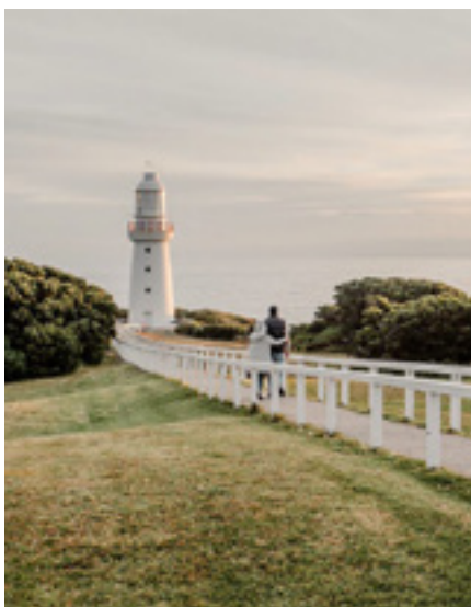
Cape Otway Lightstation is the oldest surviving lighthouse on mainland Australia and considered the most significant.
