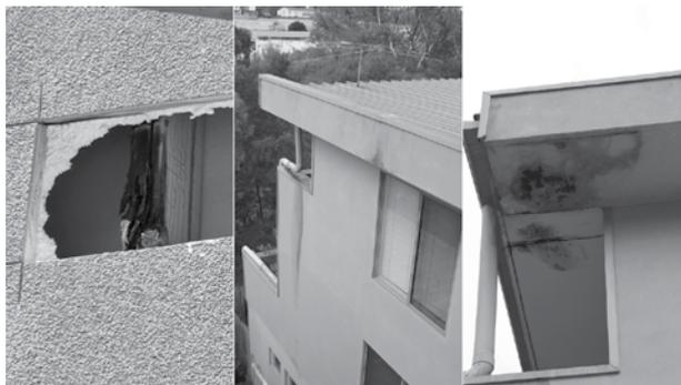
**Building A:** Evidence of water ingress and other defects. Rectification works have not yet commenced.
