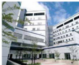
Austin Hospital Redevelopment and Mercy Hospital for Women Relocation Project
