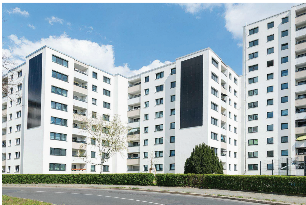
Figure 4.2 Apartment building with façade-mounted solar, Wohnpark Mariendorf, Berlin, Germany
