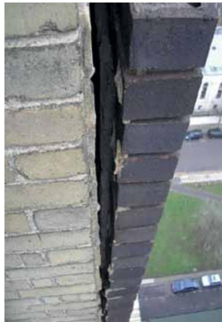
Figure 8: Brickwork in a state of disrepair and exposed concrete
