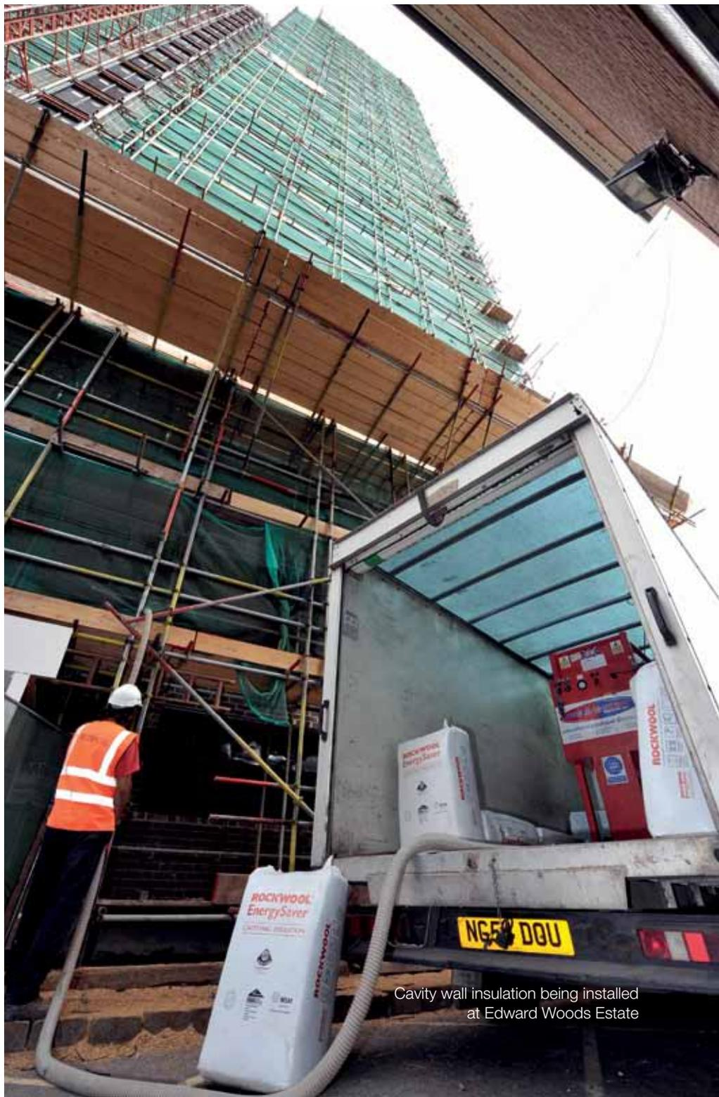
Cavity wall insulation being installed at Edward Woods Estate
