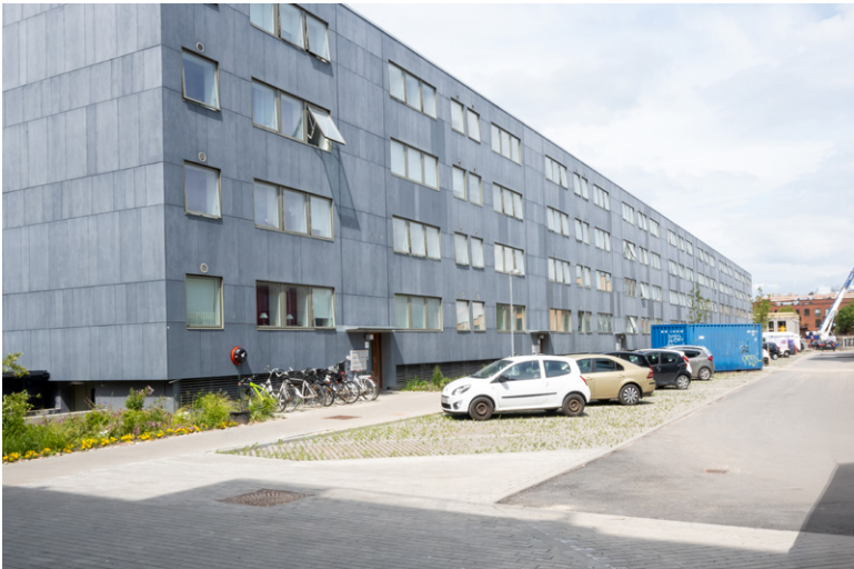
On Block 2 the facade was wrapped in cladding and insulation rather than extended with precast concrete as in the original design.
