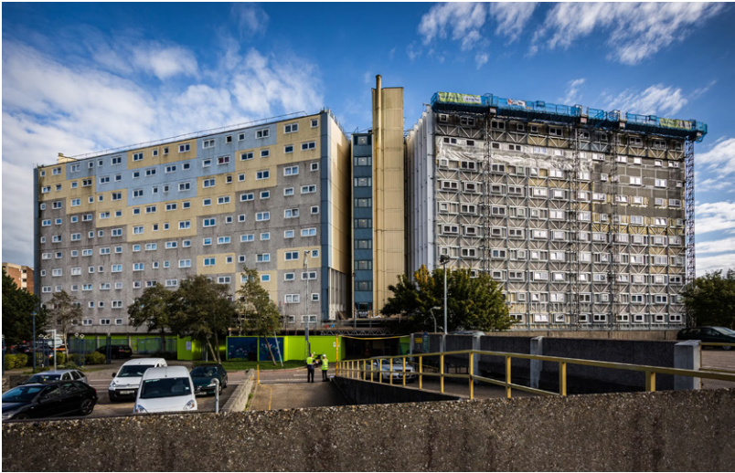
A new external facade was retrofitted to the existing concrete panels. Image from Rockwool
