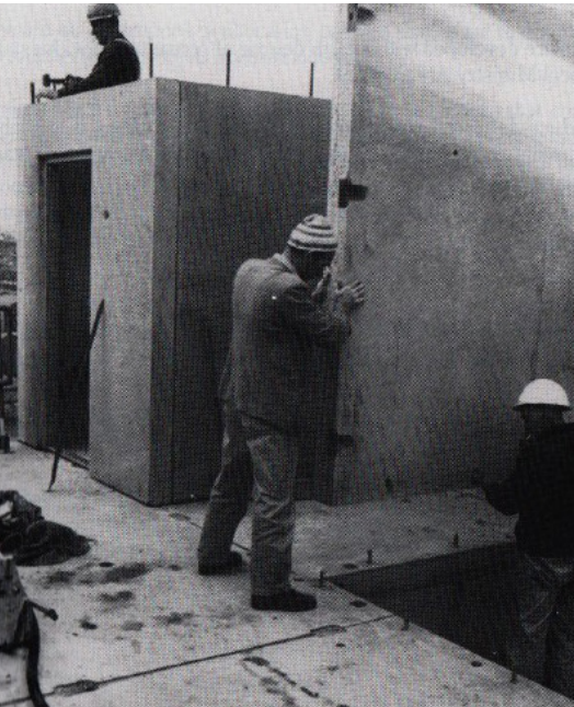
left-right. Concrete panels at the Holmesglen Factory. Placing a load bearing wall panel on site. Steel rod connectors can be seen at the top of the panel. Placement on top of the steel rods. Photos from ‘High-rise at a Glance.’
