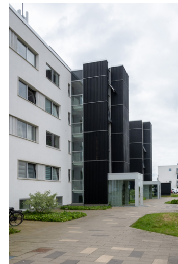
New lifts were externally retrofitted to the existing building.
