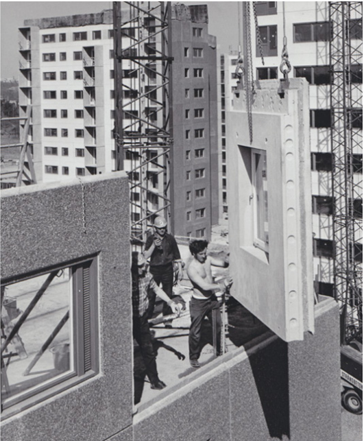
Large prefabricated panels being installed at Fittja. Image Spridd.
