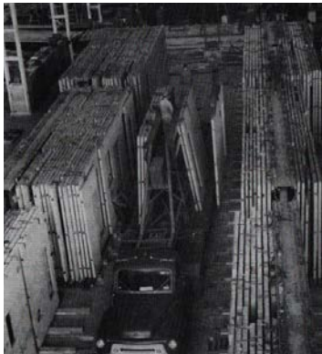
left-right. Concrete panels at the Holmesglen Factory. Placing a load bearing wall panel on site. Steel rod connectors can be seen at the top of the panel. Placement on top of the steel rods. Photos from ‘High-rise at a Glance.’
