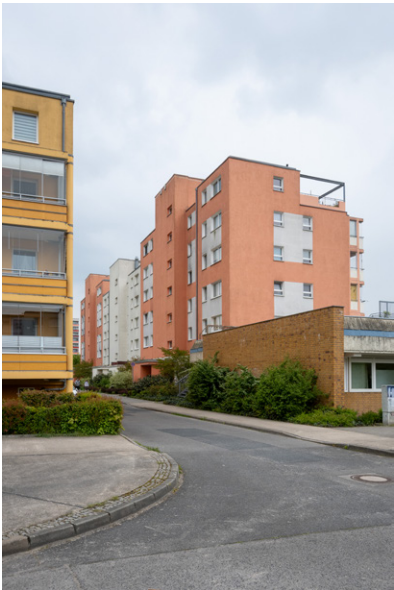
The undulating roof-line follows the modular panel dimensions as parts were removed to reduce the scale and appearance.
