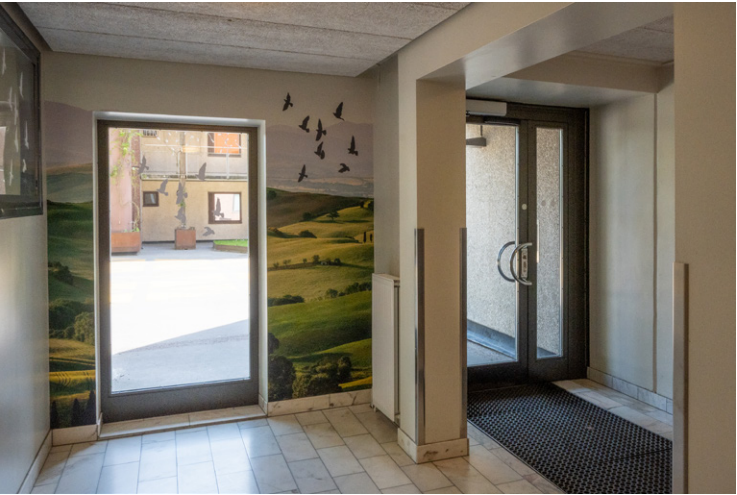
Solid doors are replaced with glazing for transparency and greater safety.
