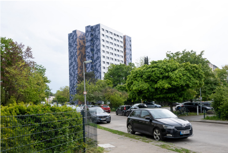
The newly refurbished tower, over-clad in a Systea composite panelling.
