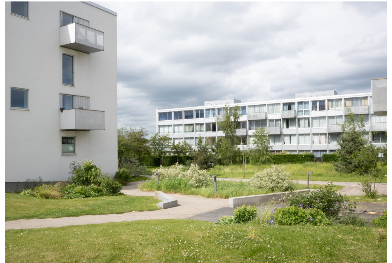
Existing building are re-clad, new openings made and balconies retrofitted.
