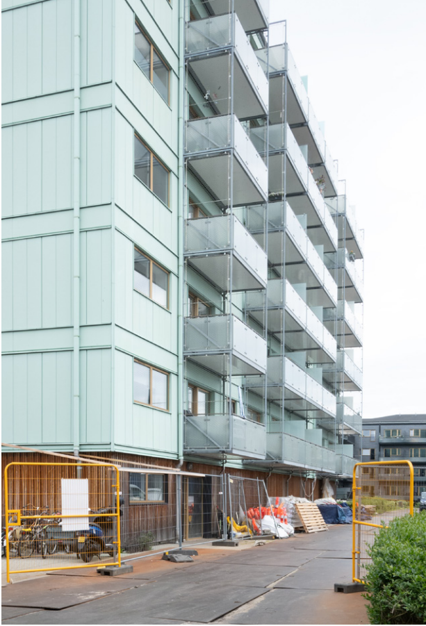
New balconies are attached and hung from the existing concrete structure.
