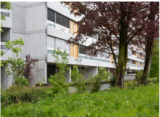
New prefabricated balconies and service risers.
