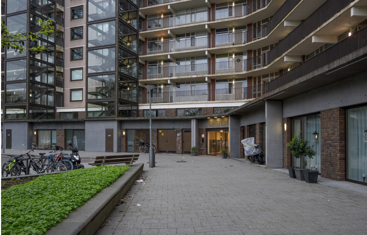
New external lifts and stairs added with the use of glazing to create a visual connection and increase safety.
