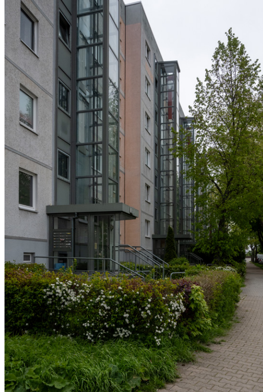
External lifts retrofitted to the existing buildings.
