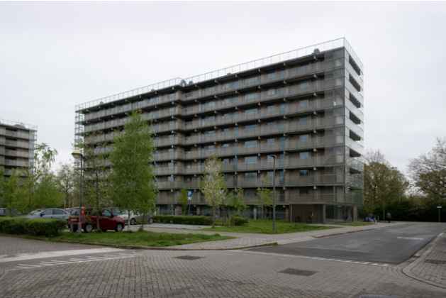
Refurbished building with new glass balustrades and facade.
