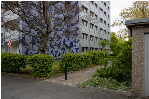
The newly refurbished tower, over-clad in a Systea composite panelling.
