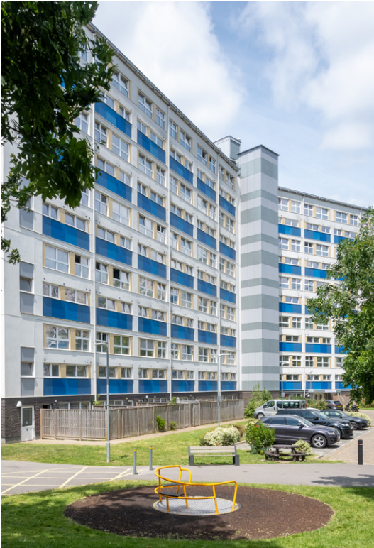
New facaded with high performance windows significantly reducing the energy demand.
