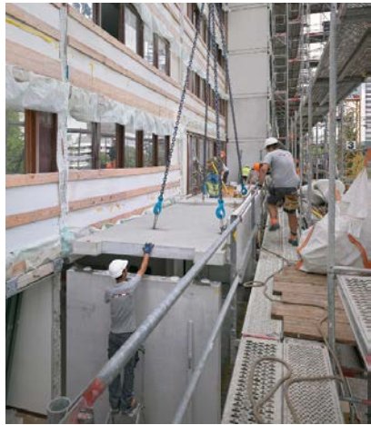
Installation of the prefabricated balconies. Photo by Fabien Schwartz, Karin Gauch
