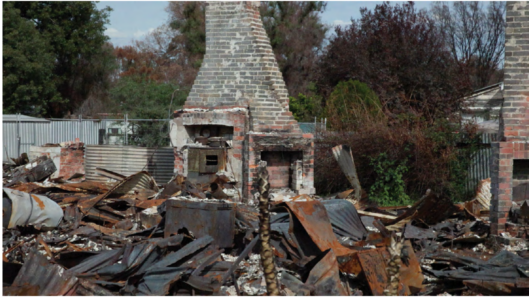
Figure 4.8 A home destroyed by fire in Natimuk
