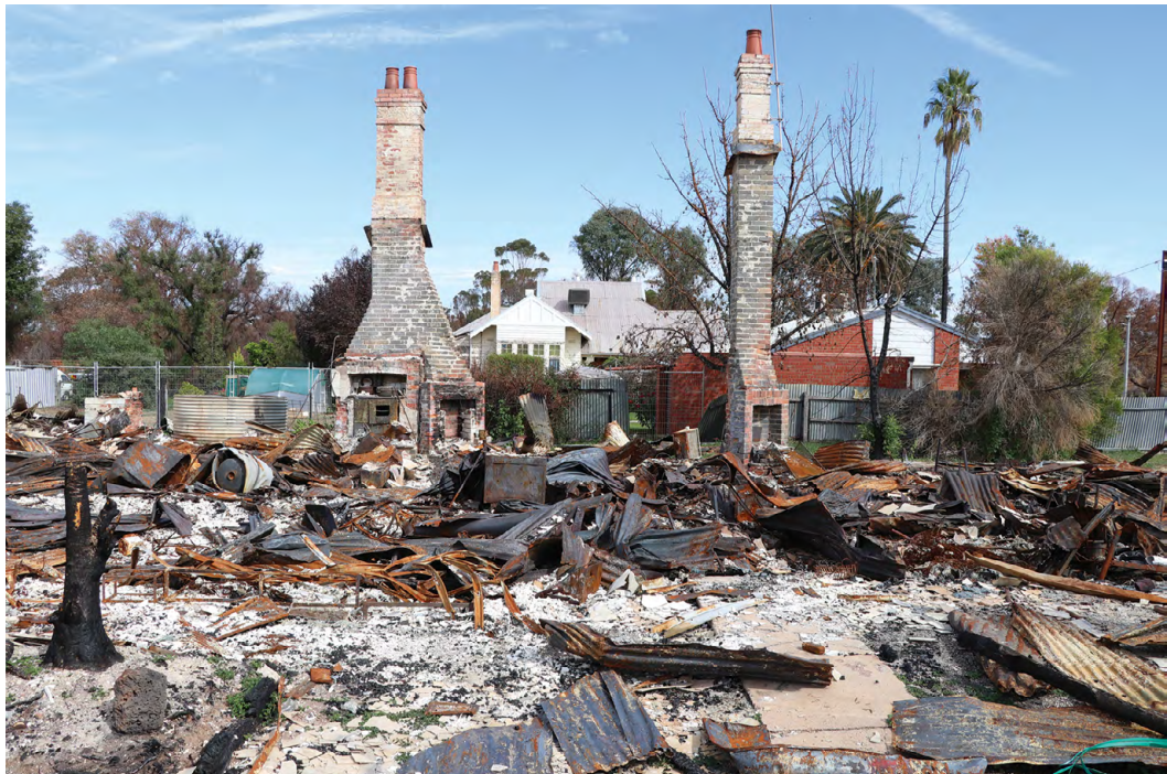
A fire damaged building in Natimuk.
