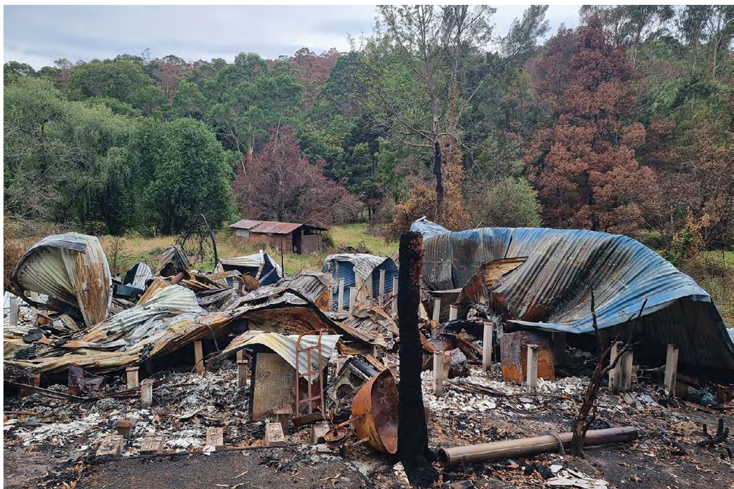
A fire damaged building in Gellibrand.
