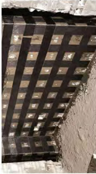
Figure 22— Example image of a concrete shear wall strengthened through the introduction of carbon fibre reinforcing in both vertical and horizontal directions.
