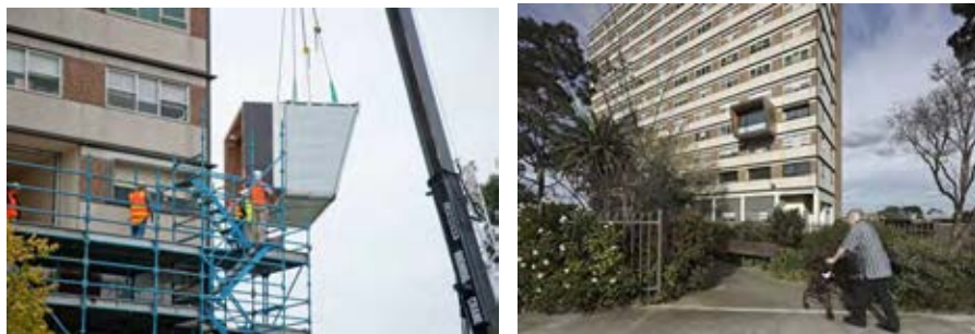
BKK's prefabricated pod being installed onto the existing high-rise building. Photo by BKK.
