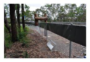
"Introducing the Fauna Escape Hatch, which prevents collisions with koalas by giving them a safe exit off the highway if they enter the corridor accidentally. The first hatches in NSW have been installed along the Hume Highway, with 8 near Wilton, at Nepean Bridge and Moolgun Creek Bridge. They're designed in line with a koala's natural instinct to push under barriers rather than climb over them, and enhance road safety for both animals and drivers."
