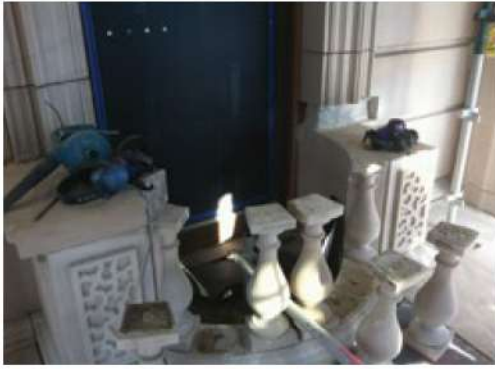
Inspection and replacement of stone balusters to the window balconies.
