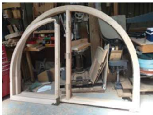
The existing hinges and corners are used where possible to preserve the history of the building.
