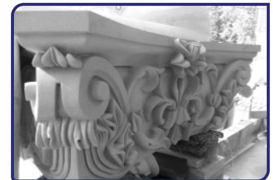
Carving of a Replacement Capital Block for Stone Restoration Works Stages three and four
