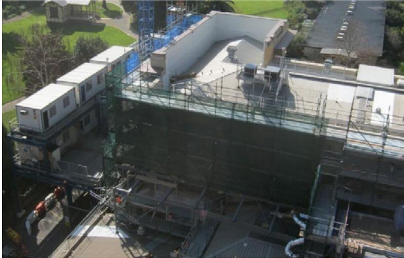
Stone Restoration Works (Stage 7): The infrastructure required to carry out the stone restoration is a significant aspect of the works including a gantry, scaffolding, lift and site sheds
