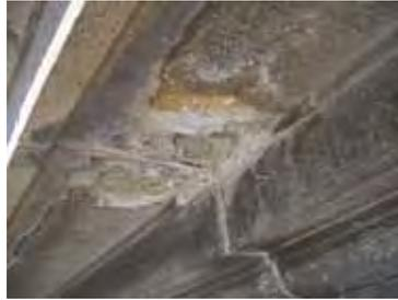
The cornice joints above Queen's Hall have deteriorated and pointing has failed. This allows moisture in to the underside of the cornice.
