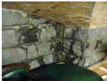
Water has penetrated the space below the front steps of Parliament House, causing extensive damage to the building interior, including Members' accommodation and storage areas.
