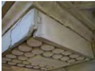
Stone restoration addresses the decay of features such as mutules and soffit carvings. The underside of these is deteriorating to the extent that a number of elements have fallen off when examined.
