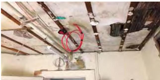
Evidence of historic and ongoing water damage to the lathe and plaster ceilings of spaces converted to Members' offices in 2011-12. These had been sheeted over with horse hair plasterboard.
