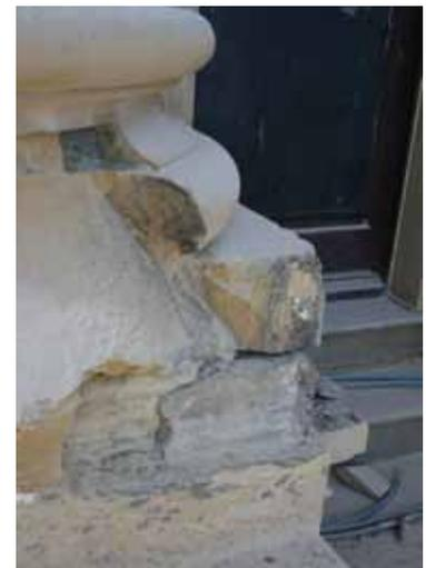
Above and below: Cracks, crumbling and deterioration to existing stone and previous repairs in library wing columns led to this stone falling away during restoration works.
