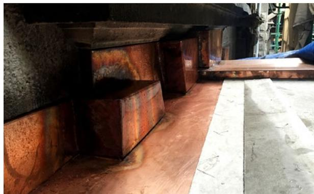
Built in the 1920's, the Billy Hughes Bridge is the timber walkway that connects the Premier's Suite with the Assembly Chamber via the existing window opening. The north facing window was removed and the facade modified to provide access and the original bluestone keystones and window header was discovered following removal of the rusting zinc flashing. A new flashing that expresses the original building fabric has been detailed and installed.
