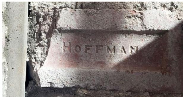
Local Hoffman bricks were used in the early stages of construction of the building and stamped bricks were found following the removal of the render.
