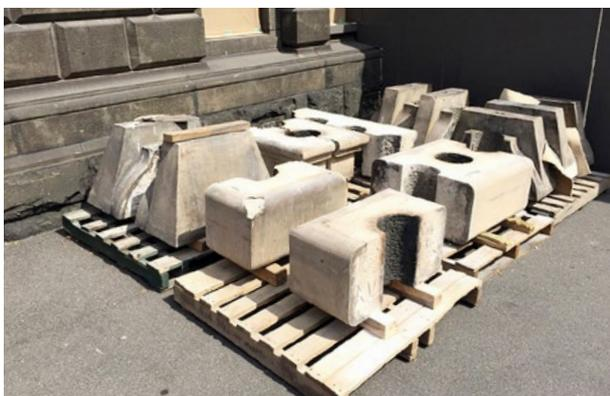
The entire chimney on the east facade was dismantled and re-laid as it was found to be leaning outward and structurally unstable.
