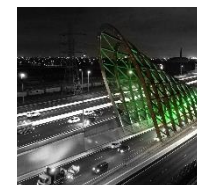
West Gate Tunnel
