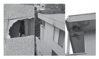
**Building A:** Evidence of water ingress and other defects. Rectification works have not yet commenced.
