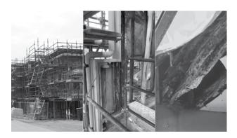
**Building B:** Cladding rectification underway in conjunction with full balcony reconstructions.
