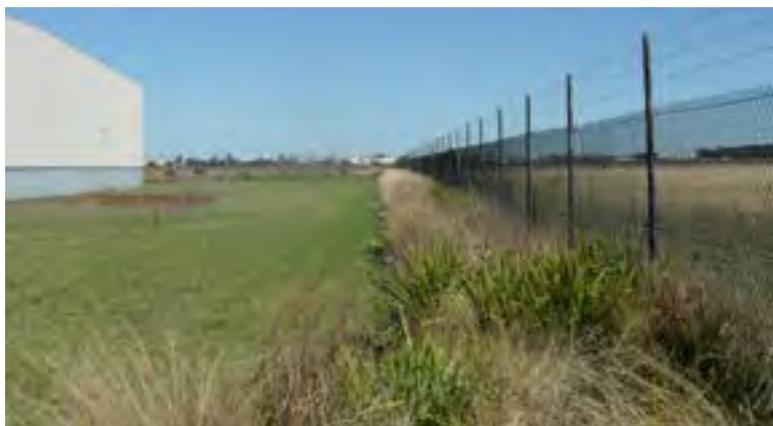
Fencing between industrial properties and grasslands will almost invariably need to provide an effective barrier to human movement. Note that barbed wire is not a wildlife-friendly fencing alternative.
