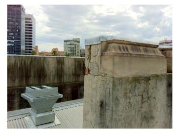
Above right: Works about to be rectified include the rear of the entire south, east and north parapet wall of the refreshments wing, rendered in cement. Cracking and moisture damage is evident with some areas of render separating from the brickwork. This is allowing ingress of water and holding pockets to form behind the render, further compounding the deterioration of the building fabric.
