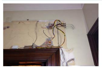
Non-compliant switchboards continue to be replaced and associated electrical infrastructure consolidated. This photo shows work in progress 29 April 2013, in a stairwell above the Legislative Council chamber.
