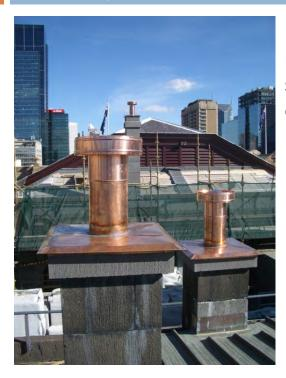
Left: A number of the bluestone chimneys on the library roof were unstable and required careful reconstruction. This required the stone masons to dismantle the chimney and rebuild them placing each stone back in its original position.
