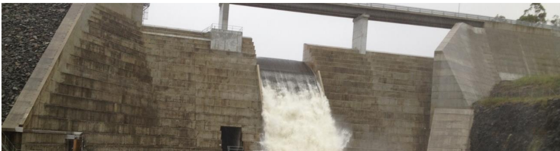
Figure 3: An example of a spillway slot – Hinze Dam in Queensland
