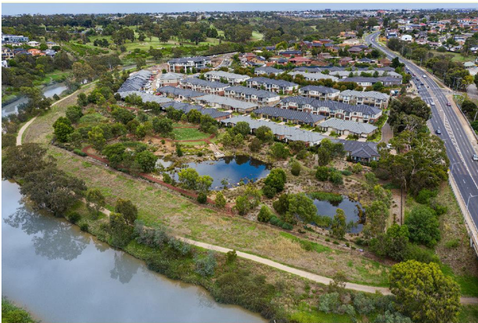
Photo of Rivervue Retirement Village, showing the constructed retarding basins in the area of the site close to the river corridor land. Canning Street is seen at the right of photo.
