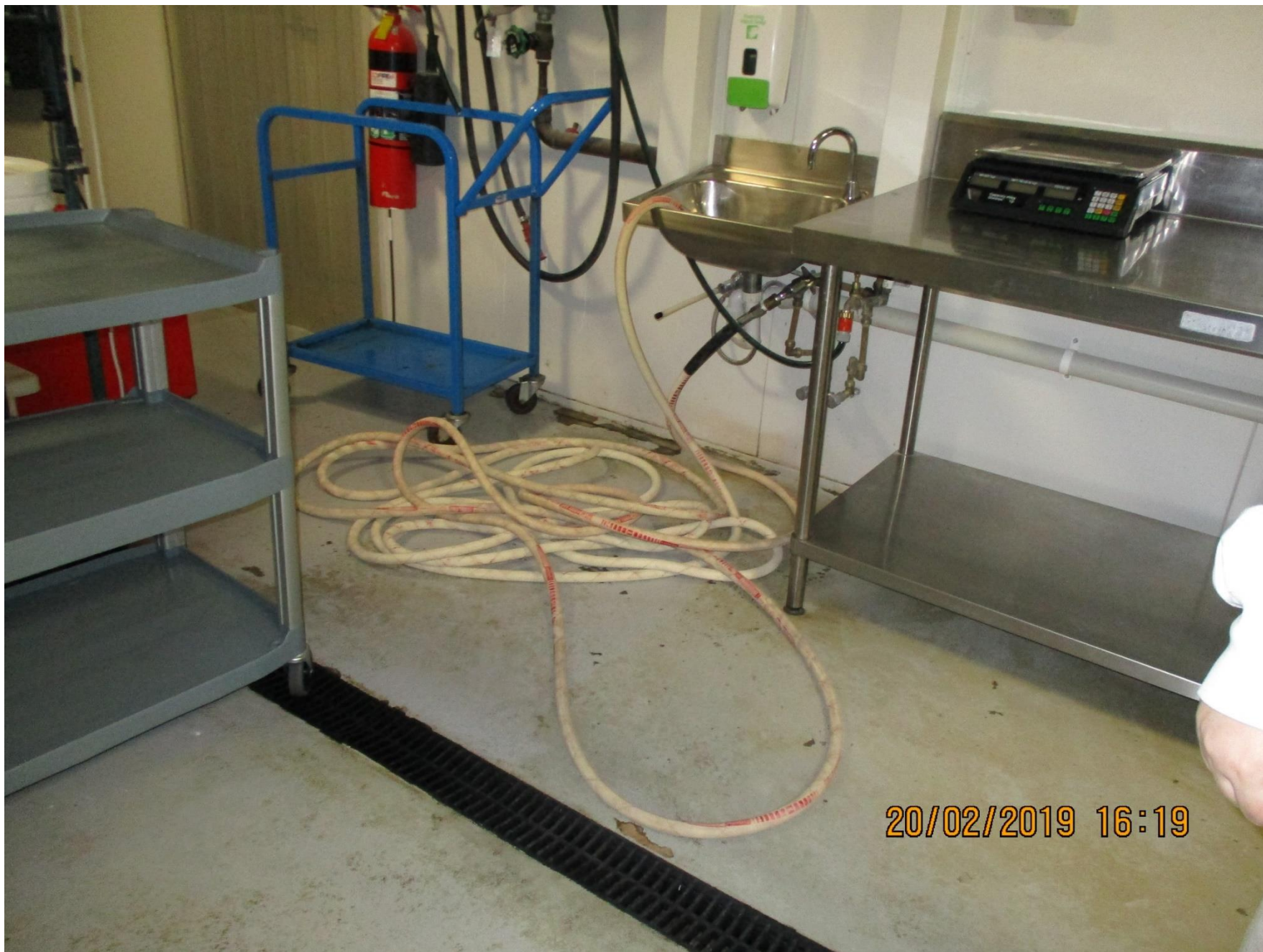
I Cook Foods – Main Kitchen photo depicts unclean floor, hose used for both cleaning and food preparation obstructing hand wash basin LJ 21
