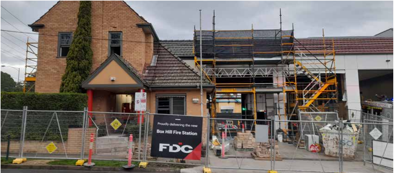
Top to bottom: Box Hill Fire Station major redevelopment.
