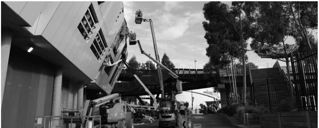
Image: Cladding rectification works on a large sporting stadium.
