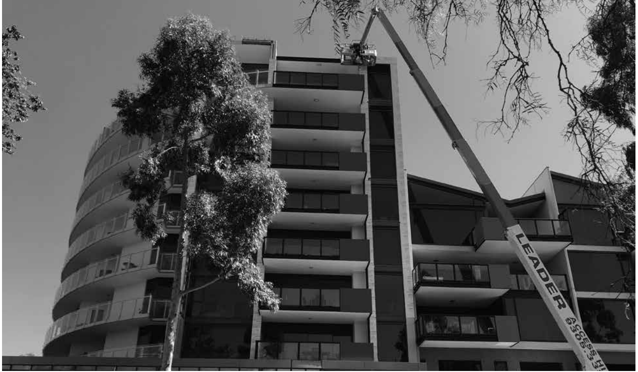
Image: A building under construction in CSV's program.
