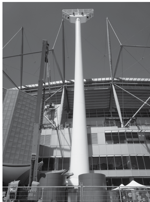
Image: Cladding rectification works on a large sporting stadium.
