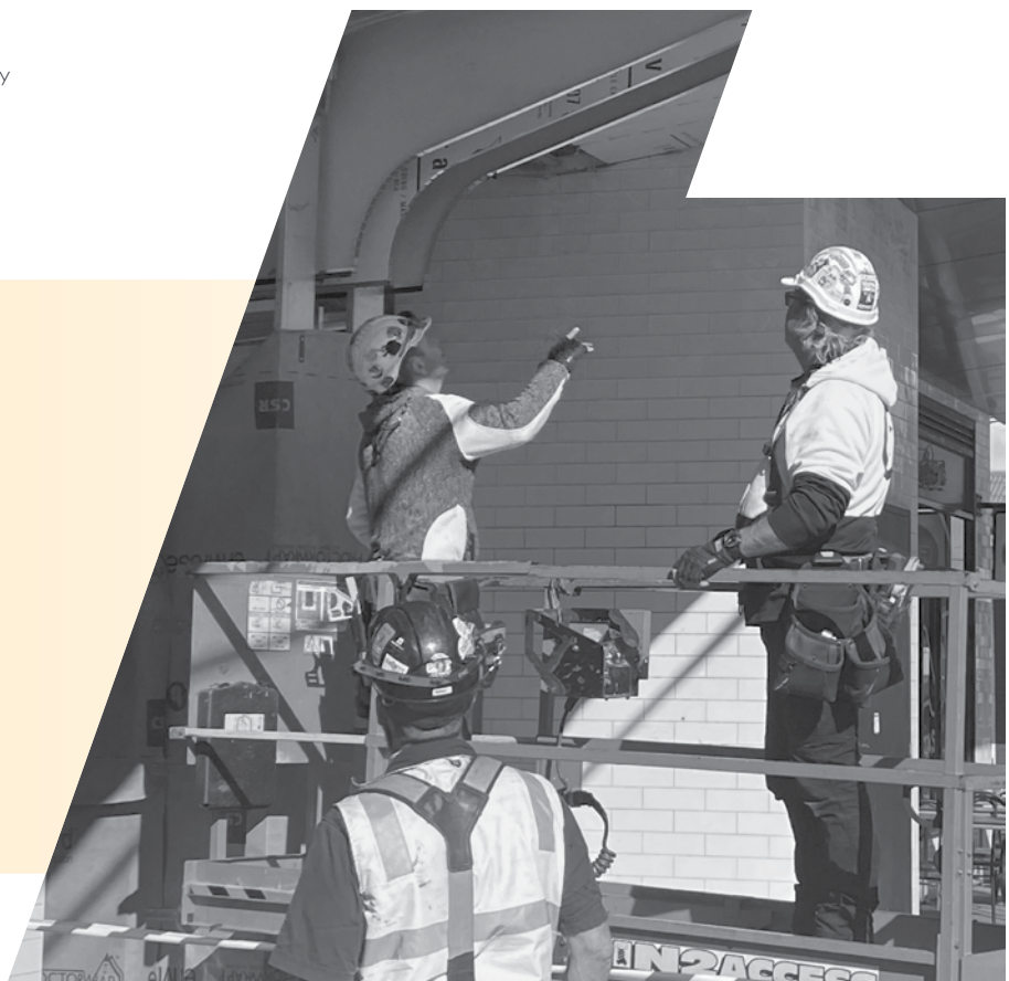
Image: A building project underway in CSV's program.
