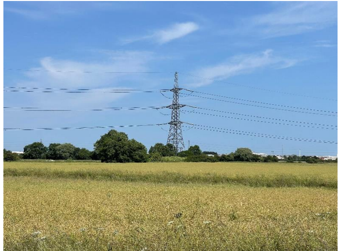
Overhead transmission lines (400kv) are prominent throughout the UK
