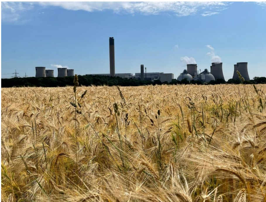
Drax Power Station co-exists with surrounding agriculture and the village of Drax literally right next door
